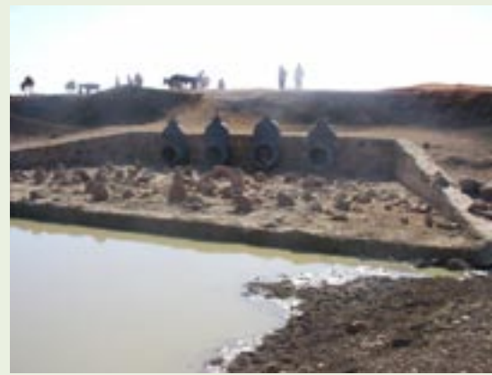
Water gates in a dam allow water to be discharged downstream in Kordofan State. For people living downstream, the dam had become a barrier to equal access to water and the gates were constructed by the Local Administration after discontent turned into conflict. Photo: Osman Abdel Rahman Alfadni, Sudan
