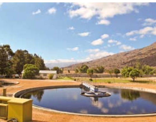
Ceres waste water treatment plant one of the six plants where Drakenstein is using the Municipal Assistant system. Photo: Dick de Jong, IRC
