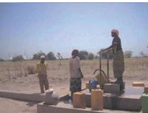
Borehole with a foot pump, visited by Group 2.
